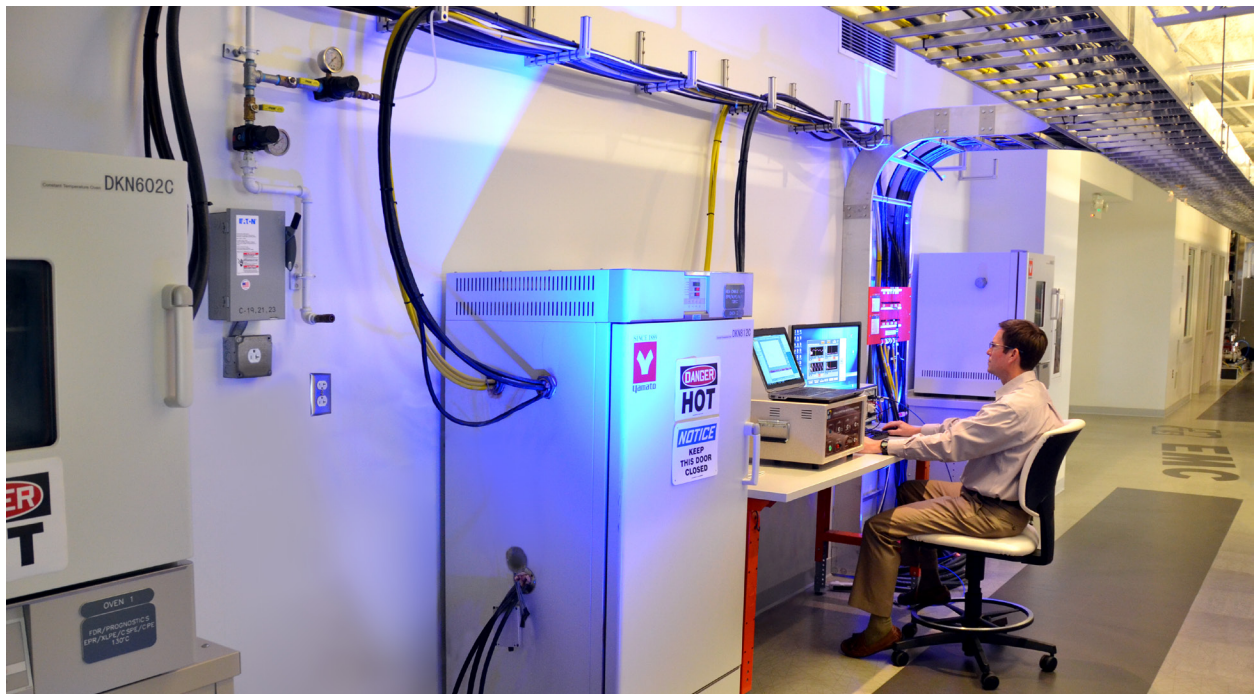
Figure 3. Cable Thermal Aging Experiments in AMS Laboratory
